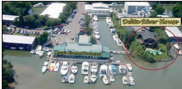
Aerial view of the Delta River House.
